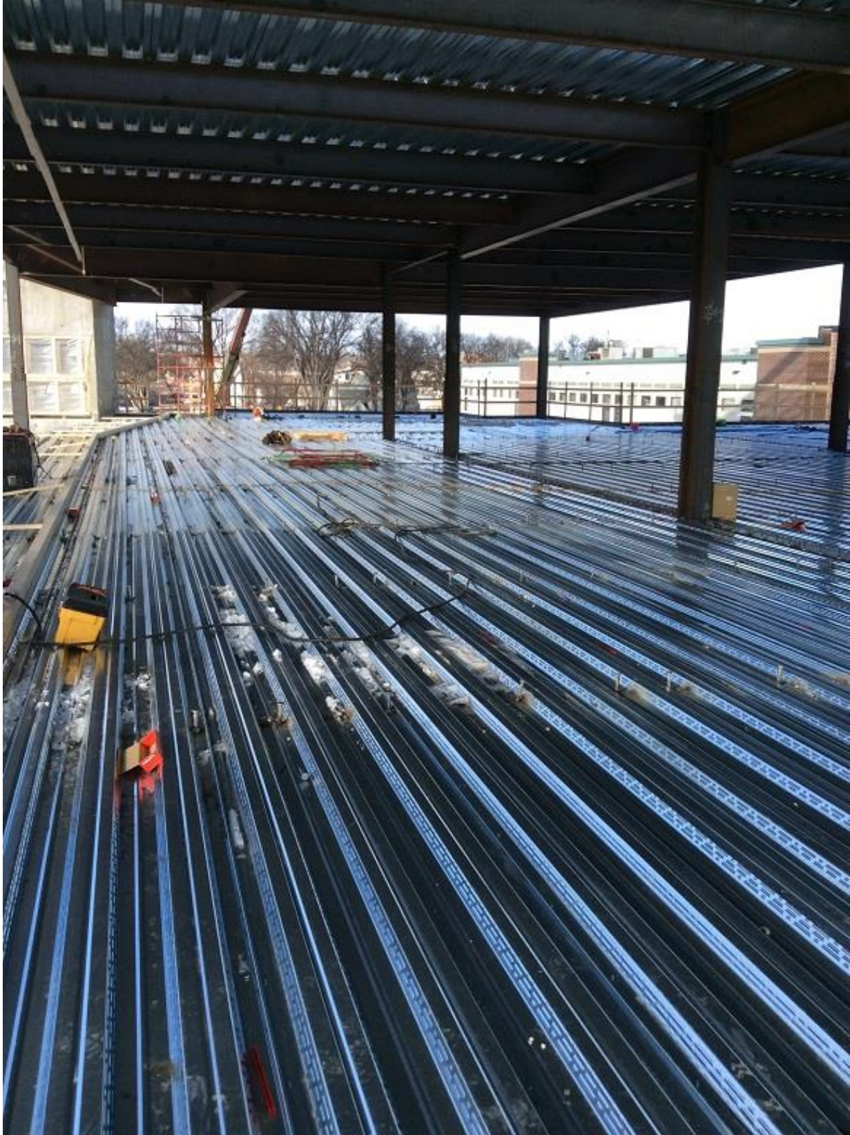
Decking Zone 1 Level 2.
