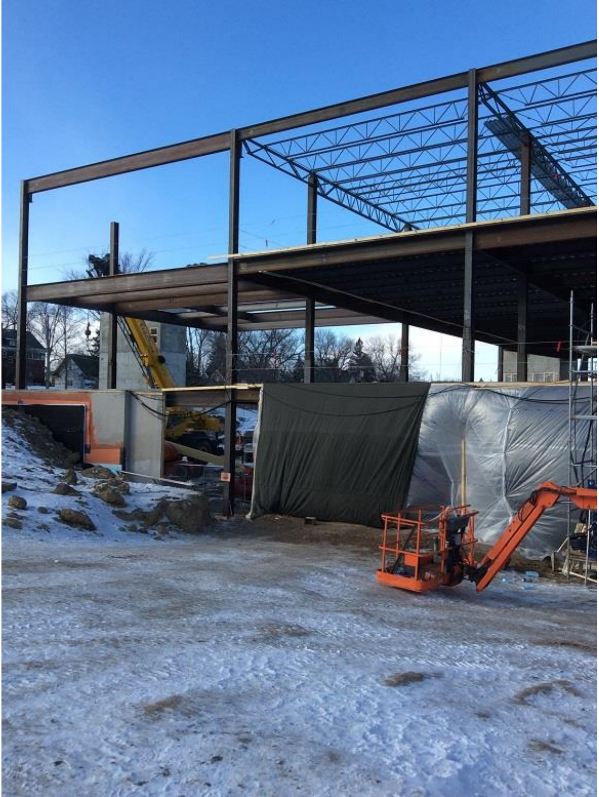
Zone 2 Steel erection beginning.
