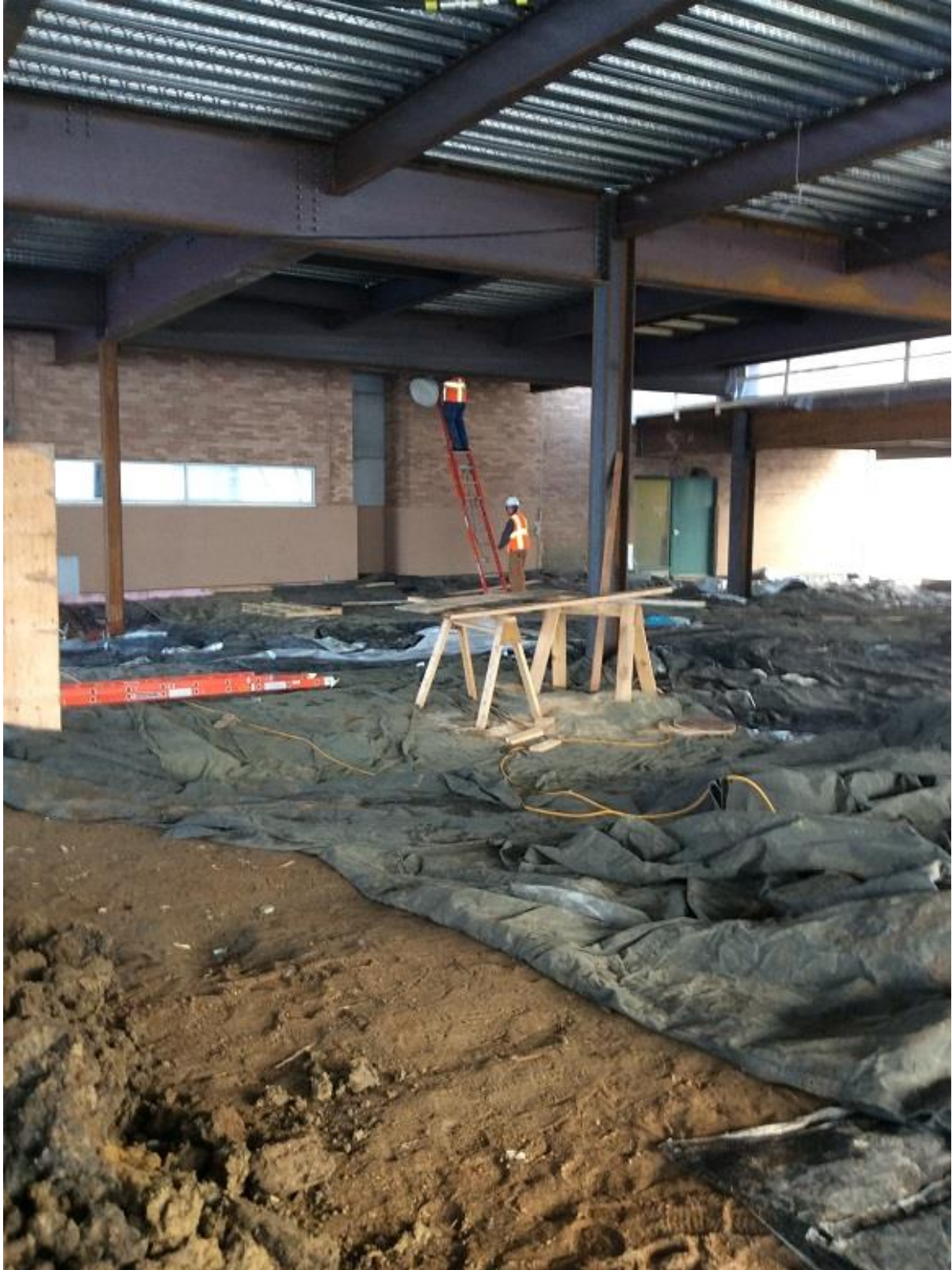
Ground heater set up in zone 1.
