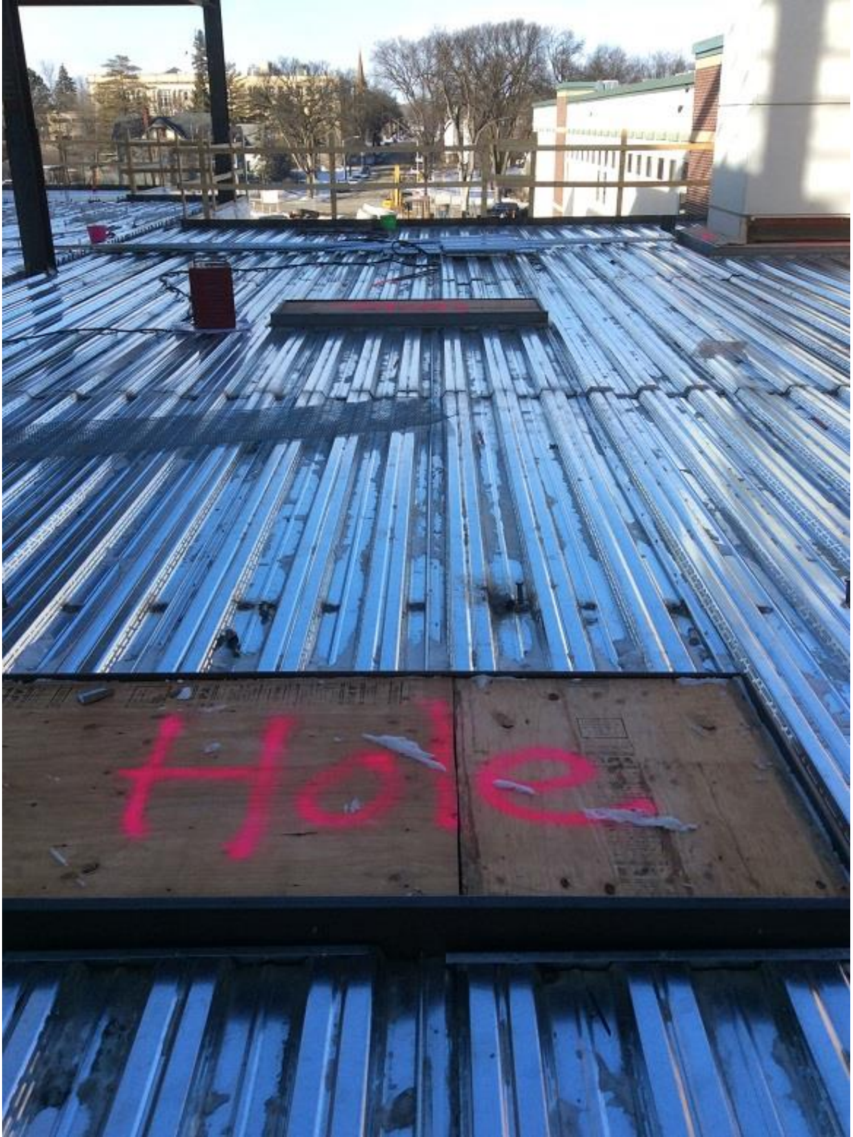
Decking Zone 1 level 3.
