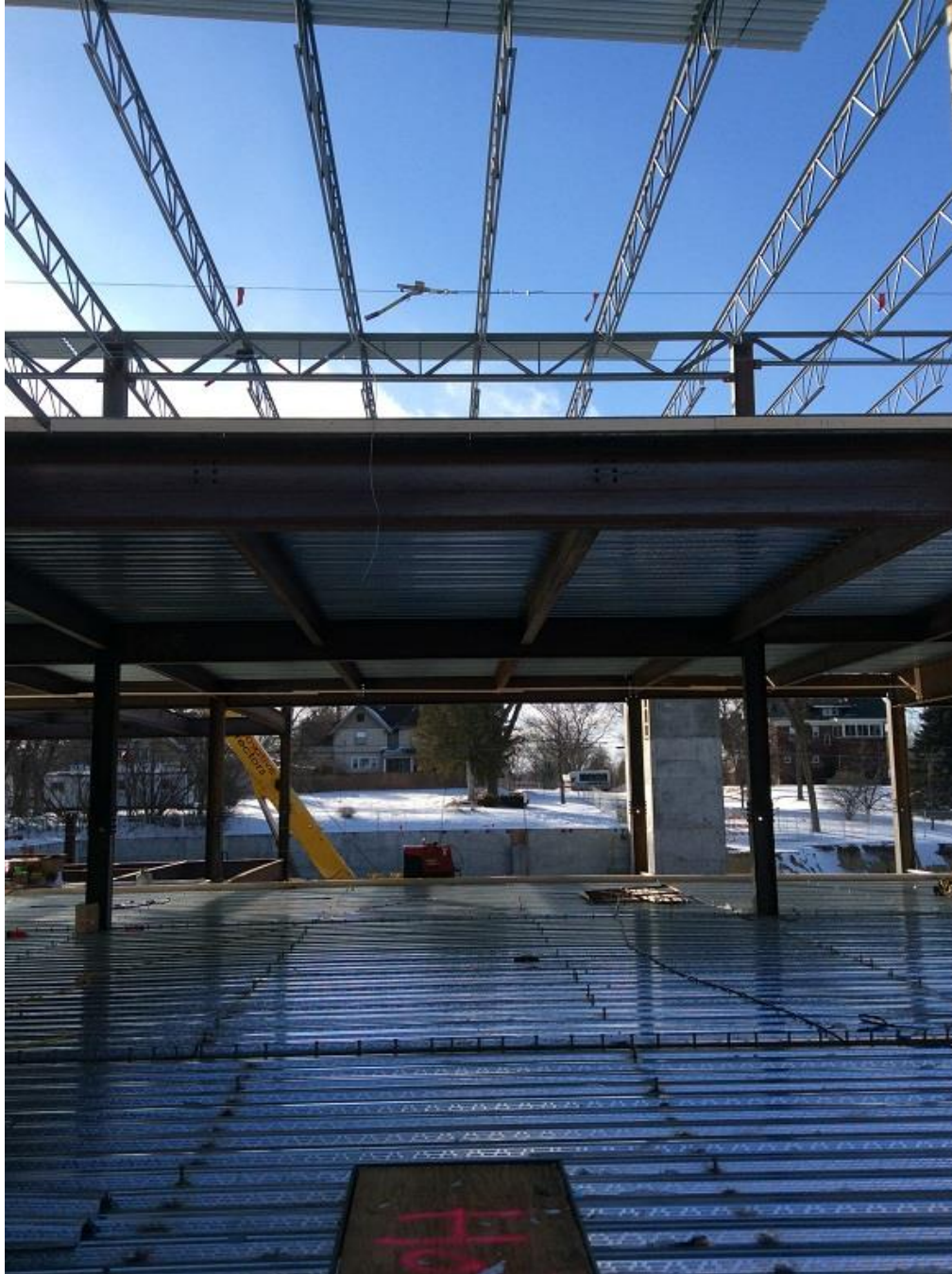
Zone 1 Level 2 Decking.
